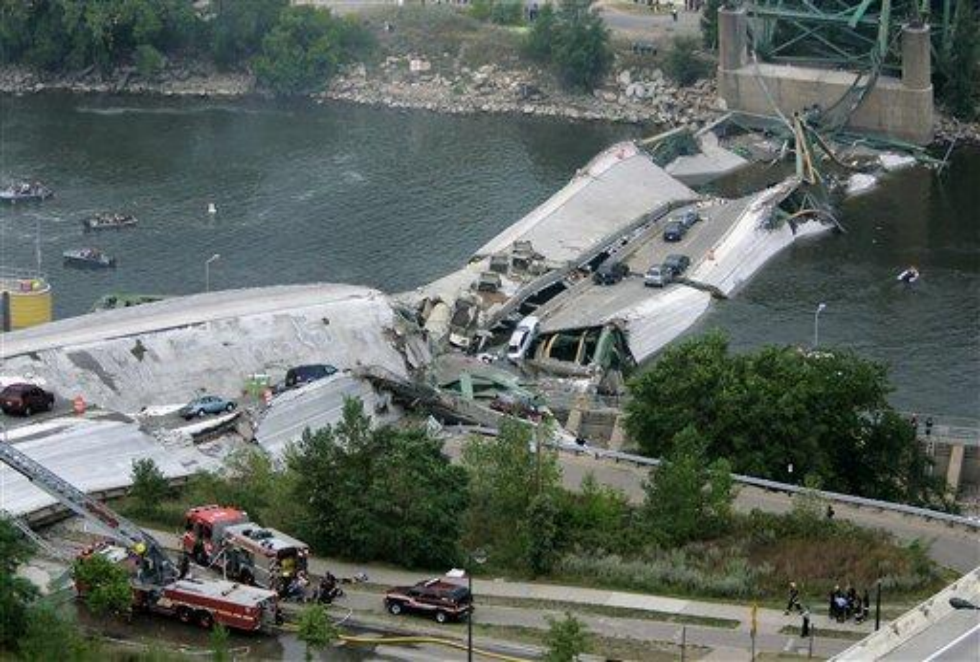
'Interstate - 35W - Freeway - Bridge' - over - 'Mississippi - River' - after - it - 'collapsed' - in - 'Minneapolis', as - 'Emergency - Crews' - 'gather'.
