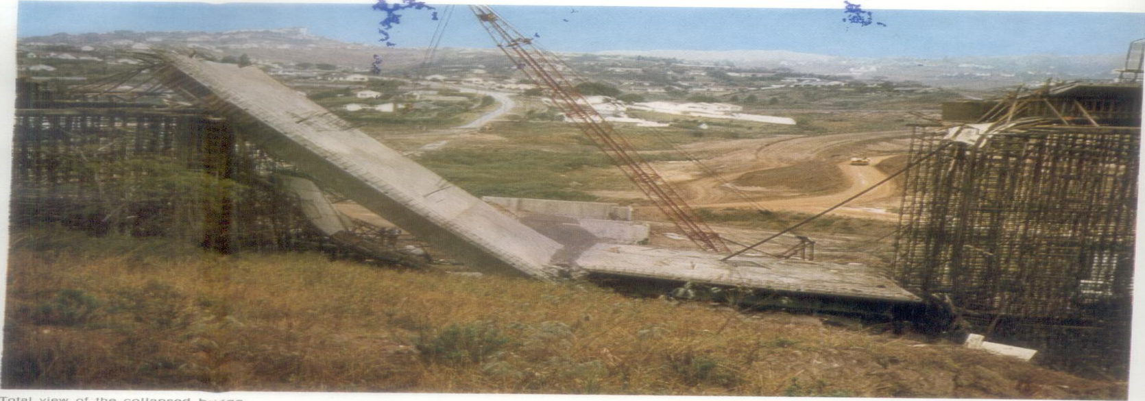
Total view of the collapsed bridge.
