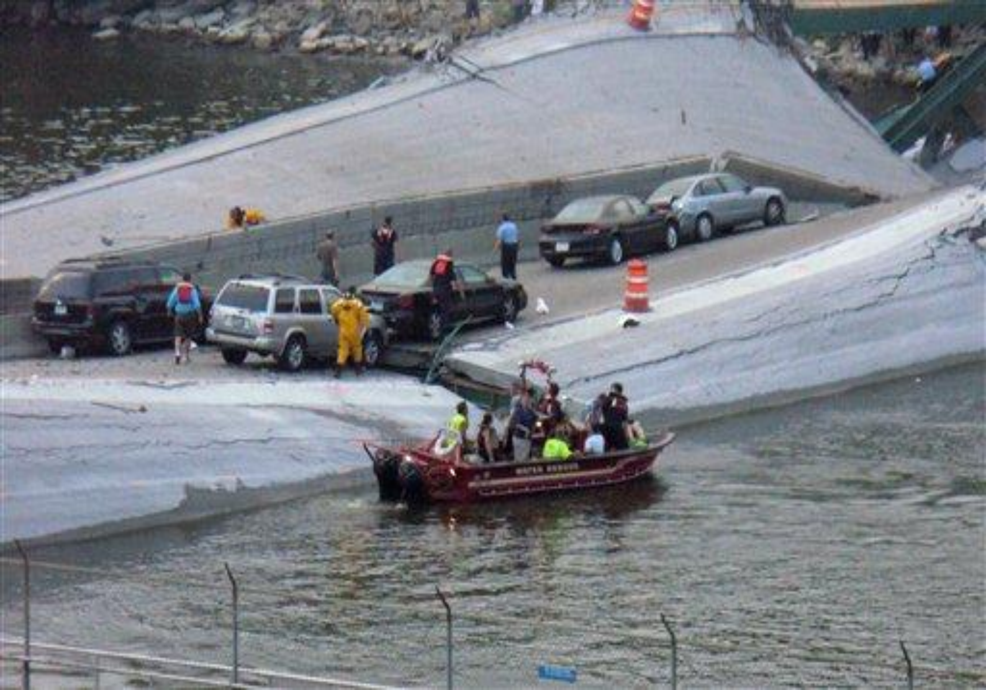
'Interstate - 35W - Freeway - Bridge' - over - 'Mississippi - River' - after - it -
