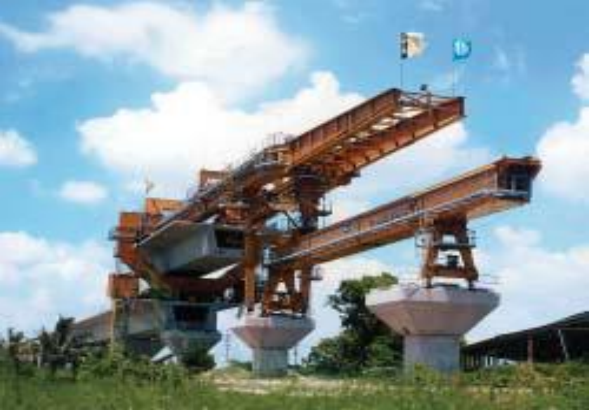
'Bridge - Launcher' - 'lifting' - a - 'Prefabricated - Bridge - Section' - into - 'Place'.
